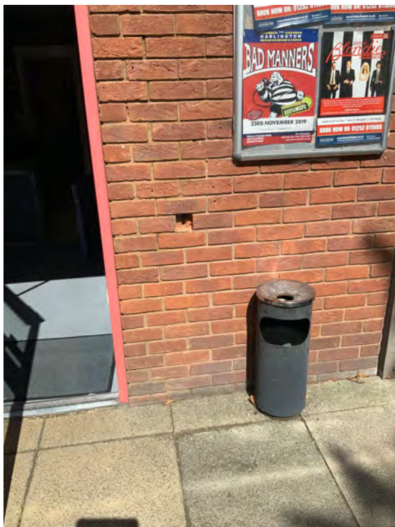
P11 Damaged brick to the right hand side of the disabled entrance door
