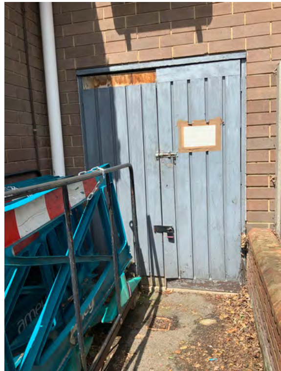
P22 Double doors to south-east elevation changing room wall. Timber cladding deteriorating.
