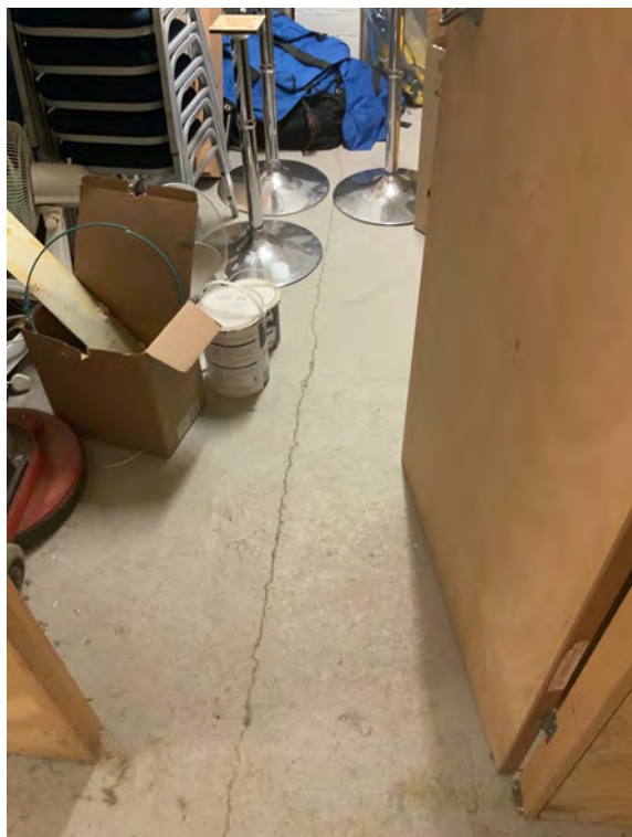
P133 Basement Store 2 – Cracked floor leading through Store 2 into the corridor
