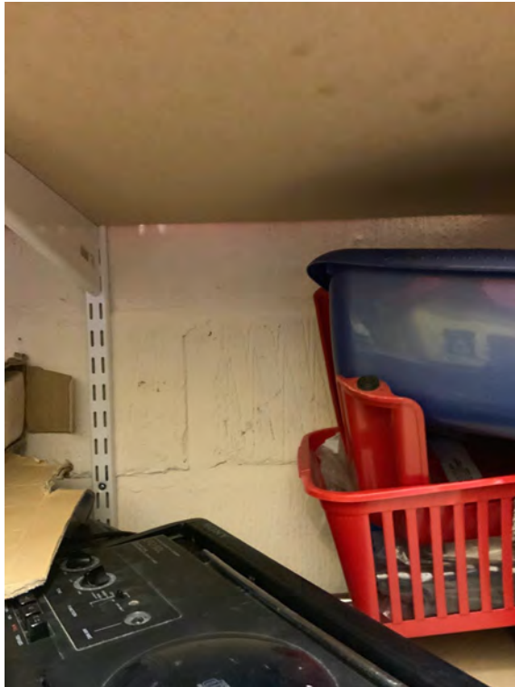
P90 First Floor, Store Behind Stairs – Cracking to blockwork joints
