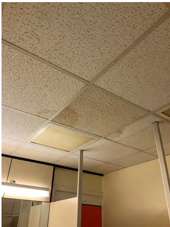
P52 Ground Floor Ladies WC – Recurring leak in ceiling
