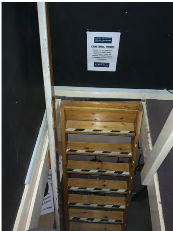
P153 Control Room Access Cupboard- No landing to top of staircase to Control Room
