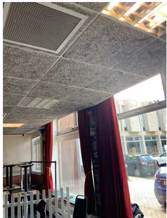
P28 Dropped area of ceiling grid to function room.
