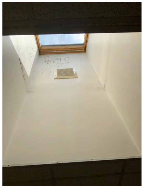
P32 Failed decoration to RVS light well in upper dining room.
