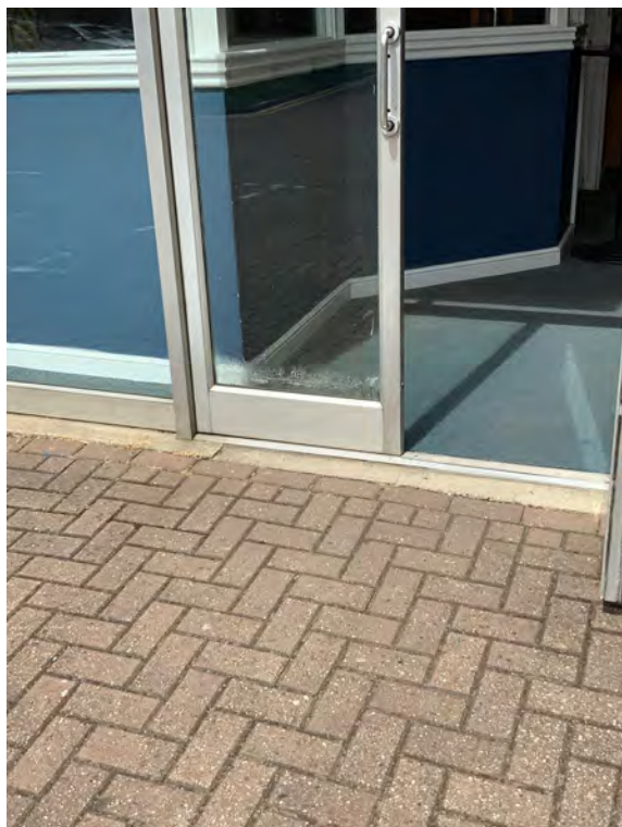
P23 South-west elevation left hand set of doors to foyer. Deterioration to bottom of left hand glazing panel
