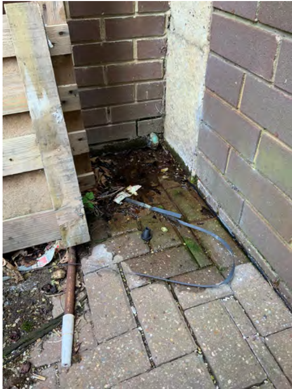
P183 East elevation, internal corner of lift enclosure. Leaking overflow pipe
