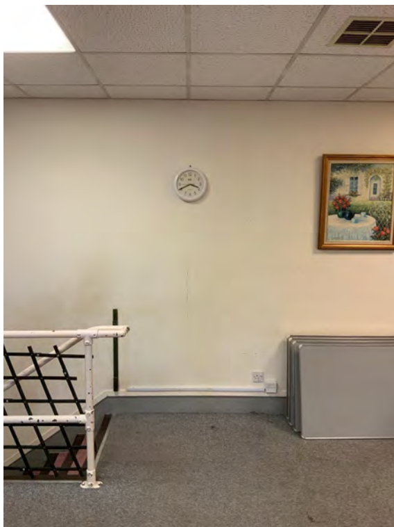
P68 RVS Main Dining Room – Vertical crack from ceiling to floor.
