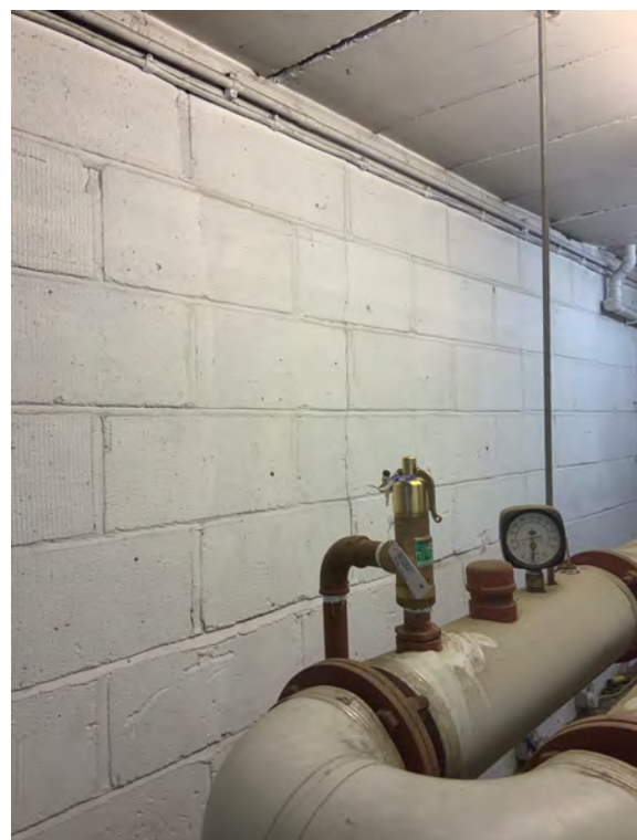
P106 Boiler Room – Hairline crack behind the boiler. These cracks are replicated at approx. 1m intervals along the wall
