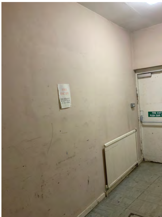
P72 Corridor from auditorium to outside – Cracking to left hand wall
