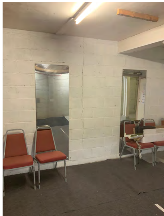
P114 Basement Stage Store – Cracks to left hand wall
