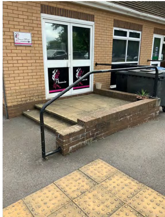
P196 North-west elevation steps to the rear of The Point. Six missing bricks and handrails would benefit from redecoration.
