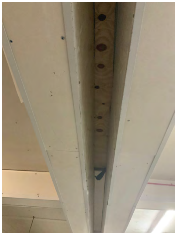
P60 Basement Stage Store – High level section of timber between beam boxing
