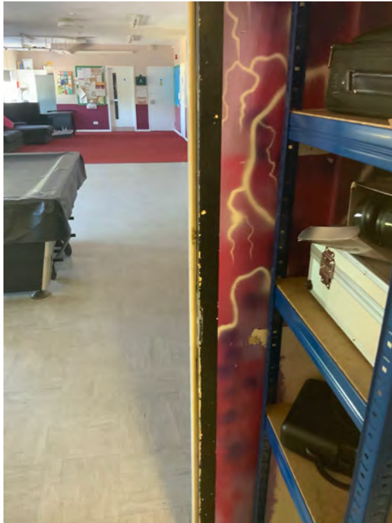
P151 The Point – Impact damage to door frame to music room
