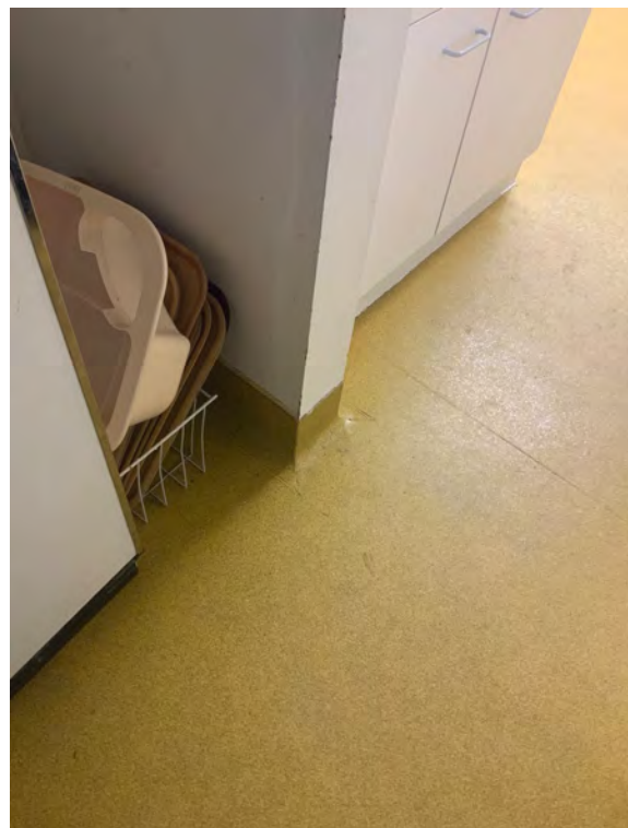
P134 Basement Freezer Room – Capping missing to floor kerb
