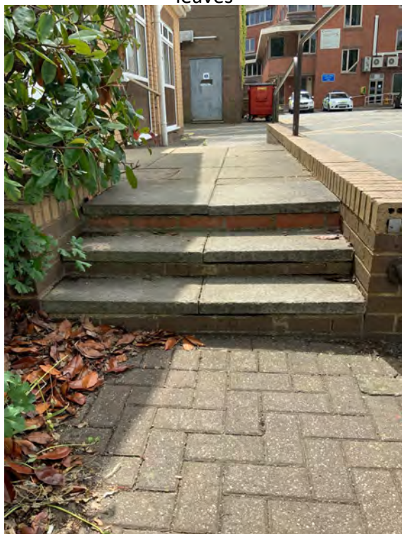
P197 Steps to RVS entrance on south elevation. Some of the bricks supporting the steps are starting to drop.
