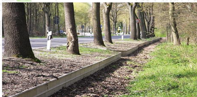
Example of road drainage to swale (shallow drainage channel for gradual water absorption)
