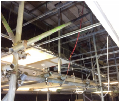
Auditorium Scaffolding: Upper Level View
