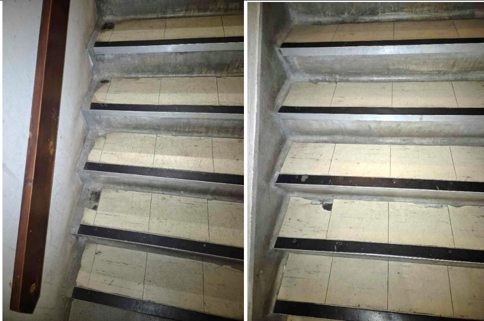
KITCHEN STAIRS – bottom (right) top (left)
