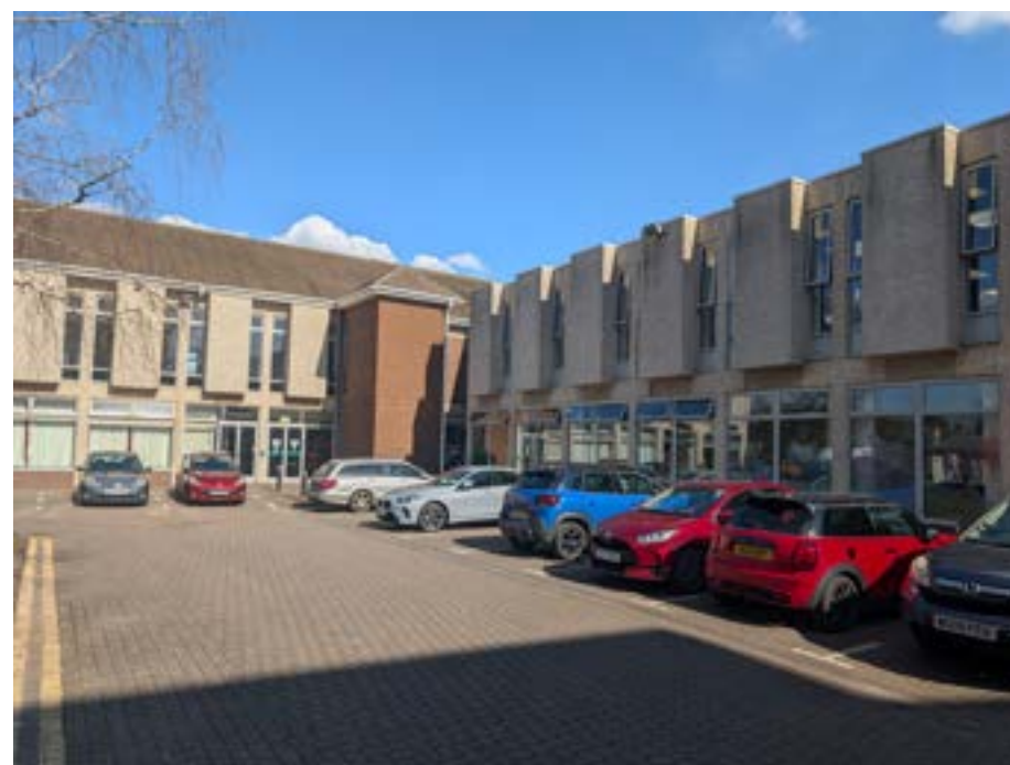
Projecting concrete bays and more recent brick lift shaft to the north-west facade of the Fleet Library facade and the south-west facade of the Harlington.
