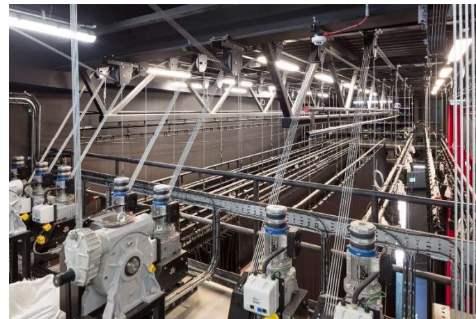
Typical pilewind hoists on a gallery adjacent to the stage
