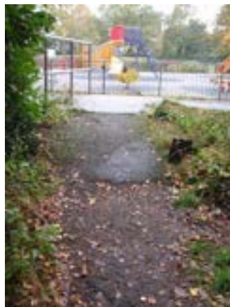
Figure 13; The section of path in need of improvements
