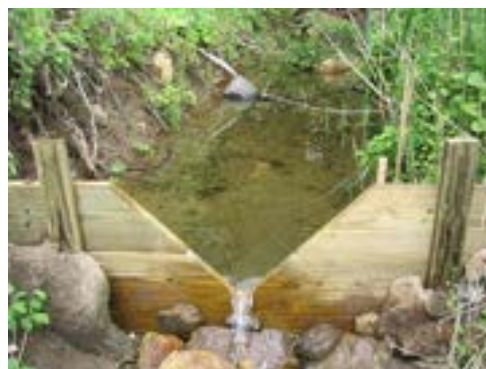
Figure 12; Example of a small notch weir
